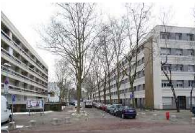
Habitat de grand ensemble Chambéry © photo ALGOE
