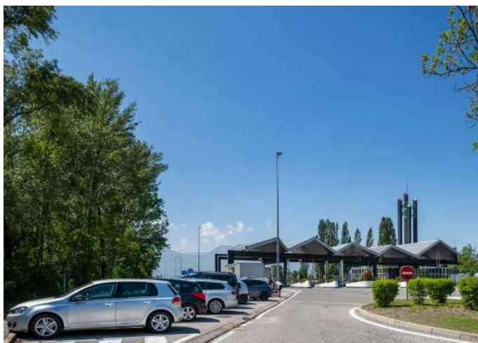
Parking relais péage autoroute Montmélian © Yannick Siegel
